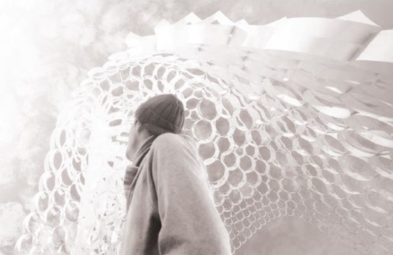
in the end, the gradient of teardrops lacked needed joints to withstand structural pressures.
